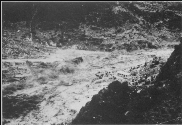
Fig 1: Flash-flood at the site of the Namche Small Hydel Plant, on August 4, 1985.
